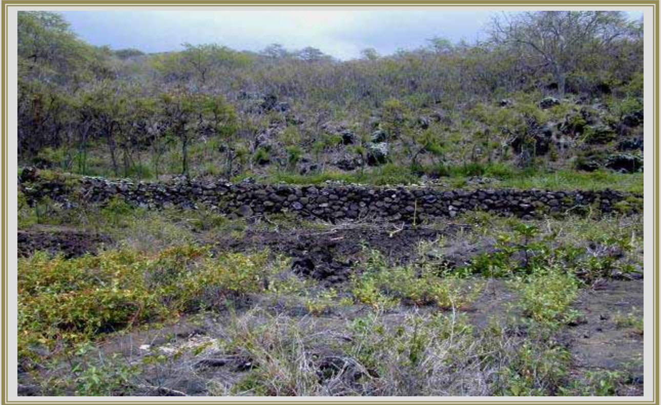
Figure 45. Makai Wall of Causeway on the Alanui Aupuni–Ka’awaloa Cart Road; Above Village on Keaweakeheka Bay near Keöpuka-Onouli Boundary (tape measure on wall is a one meter scale; KPA Photo No. 440 – August 1, 2000)
